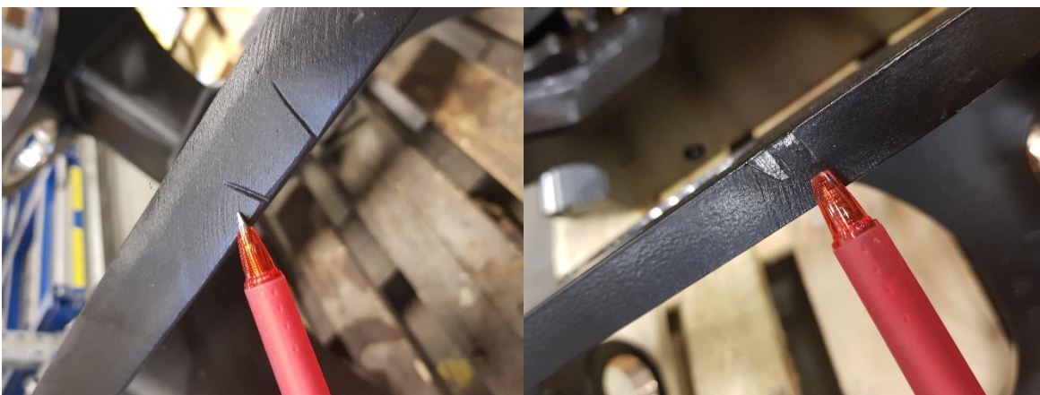
Example not permitted damages
